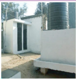
Upgraded Toilet (after intervention)
