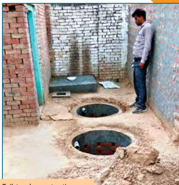
Toilet under construction
