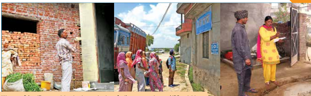
Women of the village participating in monitoring of toilet construction and IEC activities; Women volunteers involved in usage and maintenance monitoring
