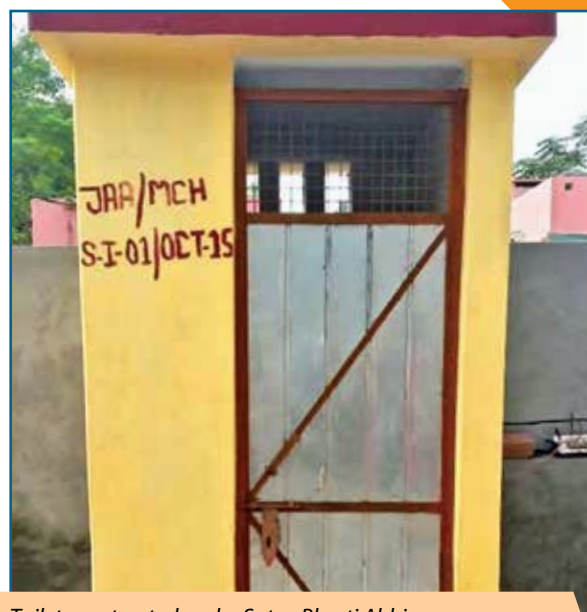
Toilet constructed under Satya Bharti Abhiyan
